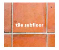
Check the subfloor for moisture problems. The joints of the SPIRIT Home 40 Click Comfort planks floor covering should never be aligned with the underlying tile joints. It is not necessary to fill the grouts of a subfloor comprised of ceramic tiles with joints when these do not exceed 5 mm in width. Bear in mind that some ceramic tiles may show rising edges/corners although the main level may be correct. These parts may telegraph through the floor covering in the future.
